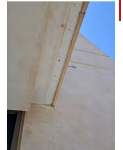
Horizontal drop around Balcony
