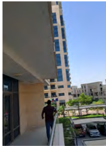
Vertical GRC Panel drop
